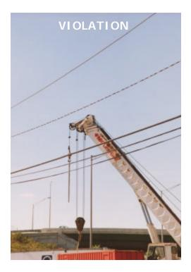
Here a mobile crane is operating dangerously close to an overhead power line. The picture shows no evidence of the lines being deenergized and visibly grounded, nor is any barrier protection installed to prevent physical contact.
