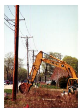
**Excavators & backhoes** are similar to drilling rigs in that they too require consideration both overhead and underground. Many types of work that requires the use of excavating equipment often take place along side of roads where power lines are present. By utilizing equipment with limited reach potential and not storing pipe, trench boxes and other material underneath power lines can reduce the likelihood of a contact.
