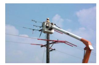
them and they must be appropriate for the type of work being performed. Workers have been electrocuted when insulating sleeves have failed and the equipment they were working with became electrified. So, never work closer than the line clearance distance.
