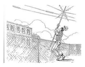
It is a concrete pump contacted overhead power lines as it was guided over a pour. Both the nozzleman, and a fellow worker who attempted to assist him, received massive electrical shocks and burns.
