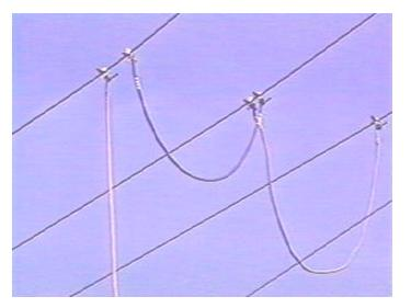
When power lines are deenergized, they must also be visibly grounded. To be sure that the lines are grounded, look for bonding cables connecting the power lines together. Two sets of bonding cables must be present, one set on each side that the crane will be working.
